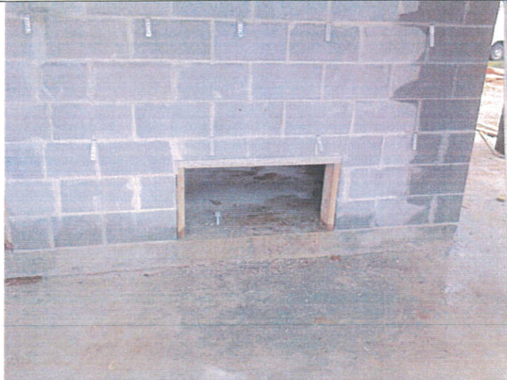
07/22/16 vent rough-in opening
