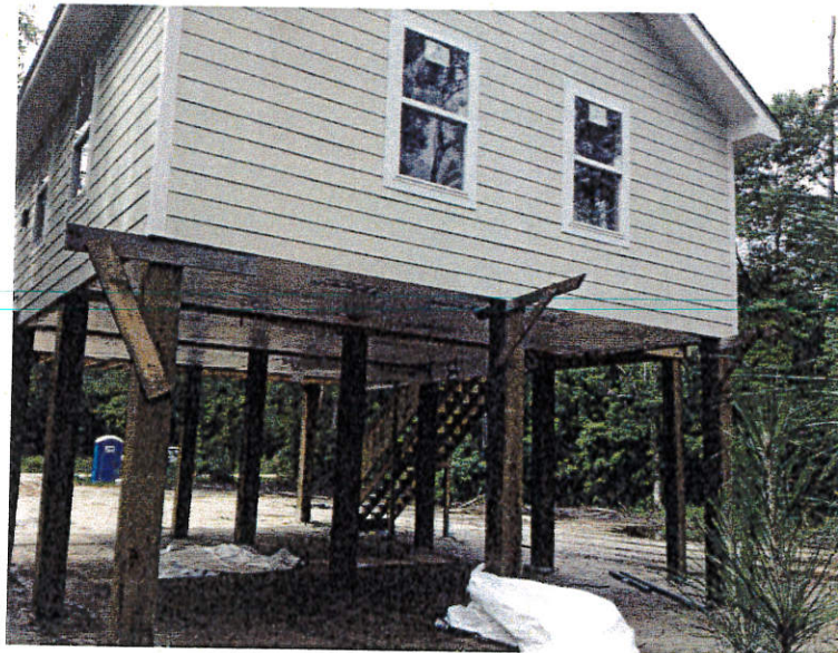
REAR VIEW OF BUILDING. PICTURE TAKEN 5/03/2013
