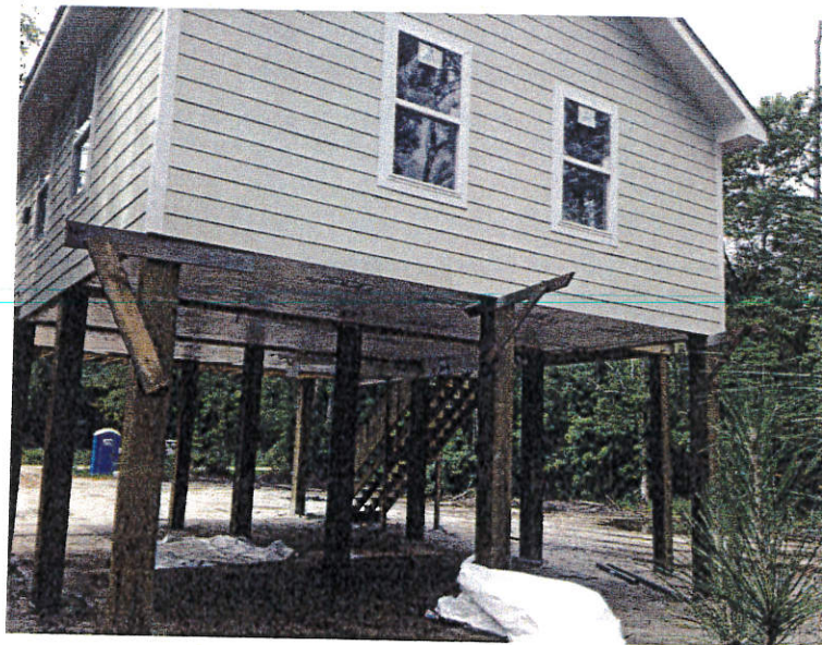
REAR VIEW OF BUILDING. PICTURE TAKEN 5/03/2013
