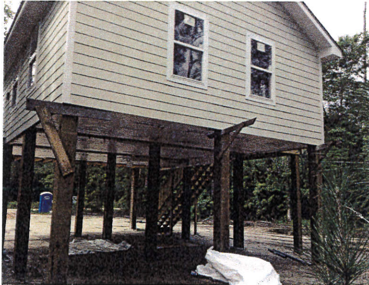
RIGHT SIDE VIEW OF BUILDING. PICTURE TAKEN 5/03/2013
