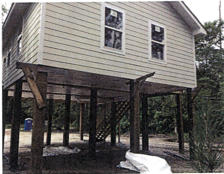
RIGHT SIDE VIEW OF BUILDING. PICTURE TAKEN 5/03/2013
