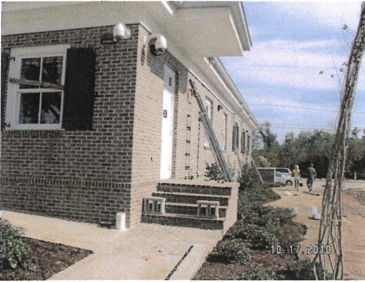
Southwest of the building looking East.
