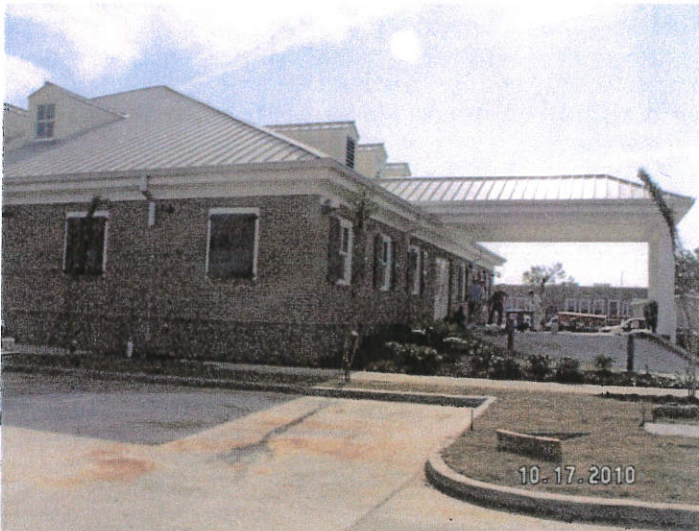
Northwest of the building looking South.
