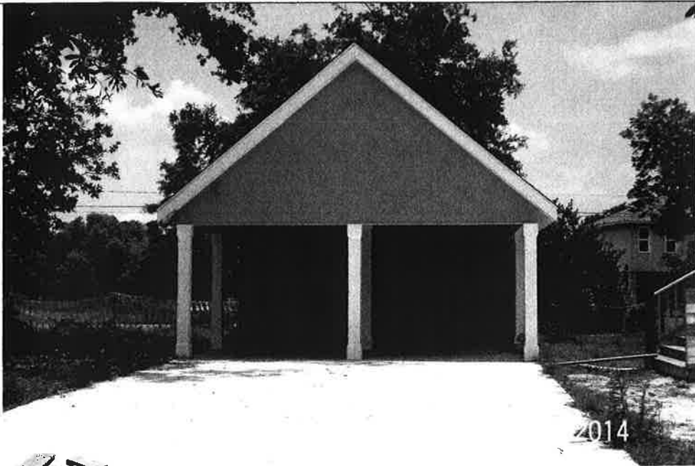
FRONT VIEW OF DETACHED CARPORT
